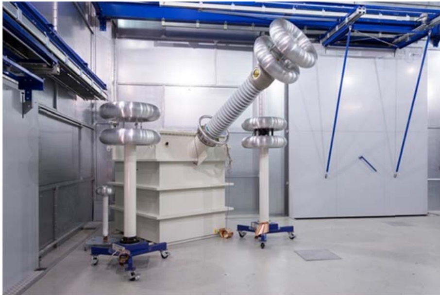
Fig. 5: AC high voltage source in the Laboratory of High voltage
