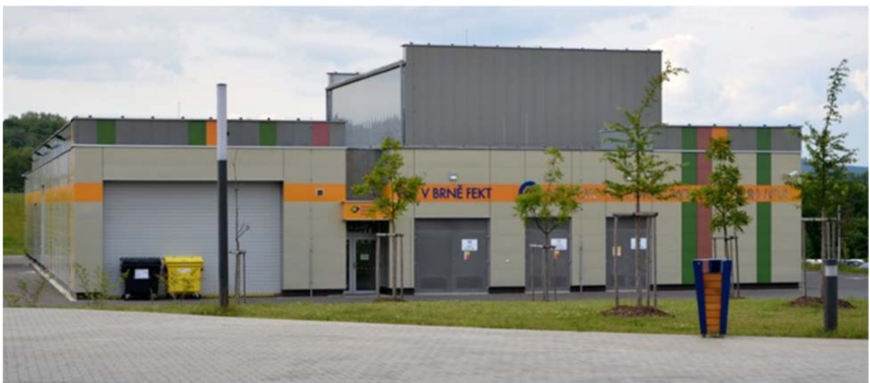
Fig. 6: External view of the CVVOZEPowerLab
